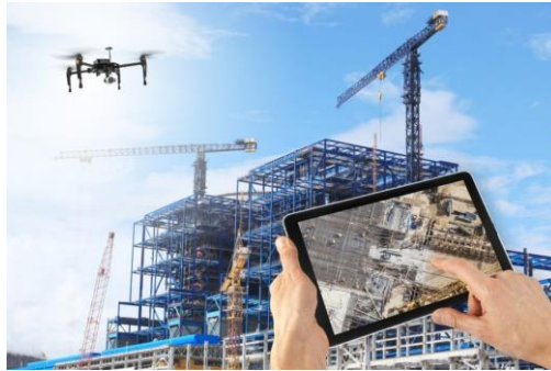
Fig1. UAV Technology in Construction site
